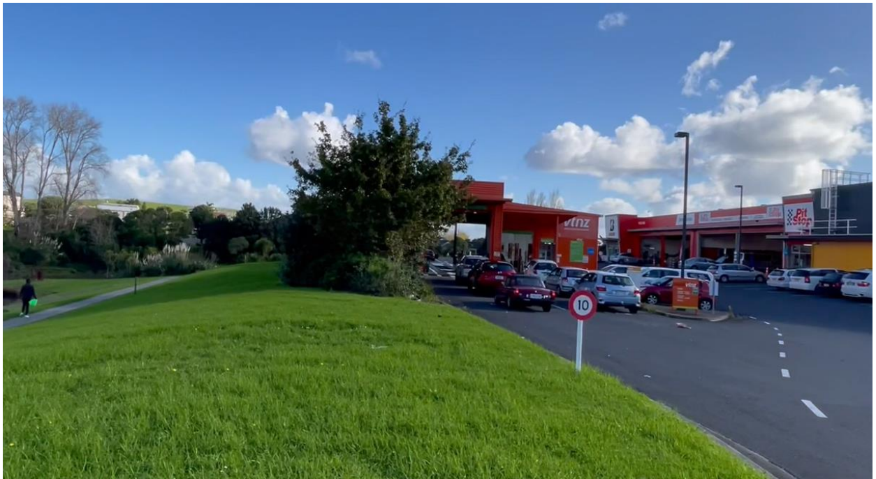
Figure 27. Location J1 – VTNZ testing station adjacent to Guys Reserve; photo taken 16 May 2023.
